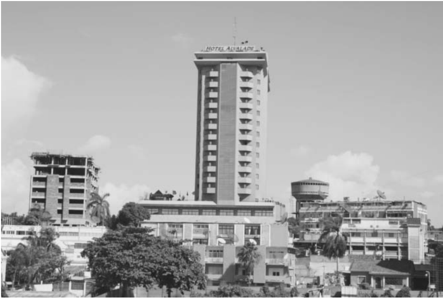
Modern urban architecture; in the middle of the picture is the five-star Hotel Alvalade in Luanda. Courtesy of Armando J. Rodriguez, Jr.
